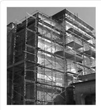
Example Frame Scaffolding (Note: This is not the actual scaffold that collapsed. Due to confidentiality, actual scaffold cannot be shown.)
