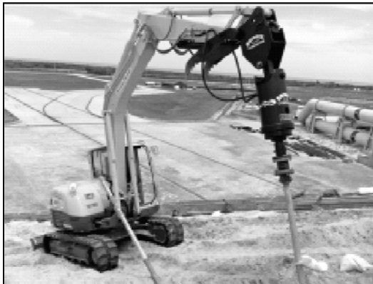
Fig. 1 Installation of Helical Piles at NASA Launch Pad 39B
