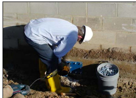
Fig. 10 Bracket Installation
