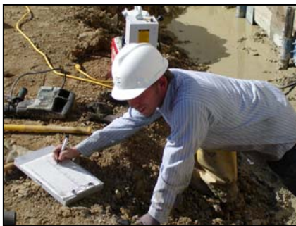
Fig. 12 Logging Pier Depth and Hydraulic Pressure
