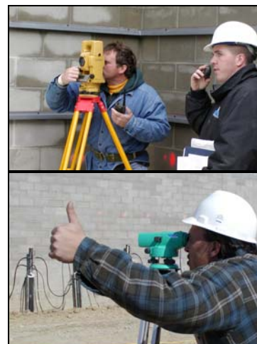
Fig. 13 Monitoring Wall Movement During Lifting Phase
