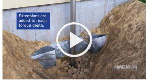
Underpinning conducted with helical piles, a lifting assembly and a ram kit to stabilize or lift a foundation.
