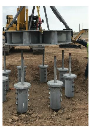
The project installed numerous all steel foundations for power transmission poles in very remote site locations. The all steel foundations provided flexible construction methods and provided a cost effective solution compared to other foundation designs.
