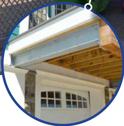
Deck And Balconies
