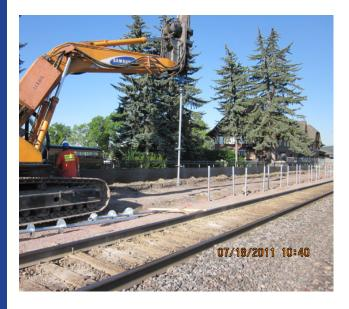
Amtrak reconstructed each of the 5 stations by adding concrete platforms for a safer and more convenient loading and unloading area for pedestrians. Original plans called for drilled concrete piers, however, due to contaminated soils, inability to shore live tracks while drilling and limited areas for oversized drill equipment, drilled concrete Over 500 MH325BR-25 ton helical piles were installed across 5 different Amtrak stations
