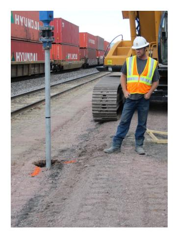
Helical piles were selected because no soil spoils are produced, no excavation or shoring was needed for the tracks, the tracks did not have to be shut down, limited access equipment and less manual labor around live tracks was a benefit. The projects were successfully completed on time and under budget.
