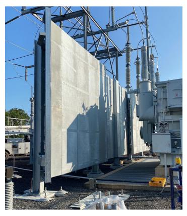
substation. Over 150 linear feet of the 20' tall blast wall was supported on the Magnum foundation system. The wall layout consisted of 12 helical pile supported columns & 5 concrete supported columns.
