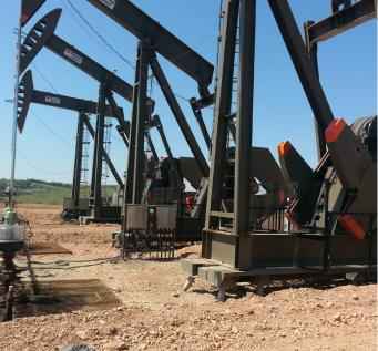
Case history utilizing Magnum foundation products for support of oil pumping units on helical piles with unique steel mat foundation elevated above gradeHelical piles were selected because no soil spoils are produced, no excavation or shoring was needed for the tracks, the tracks did not have to be shut down, limited access equipment and less manual labor around live tracks was a benefit. The projects were successfully completed on time and under budget.
